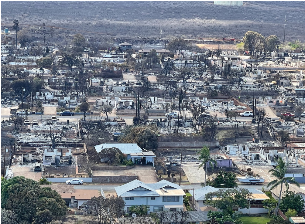
Aerial photos of Lahaina (West Maui) after the wildfires. Credit: Hawaii Department of Land and Natural Resources
