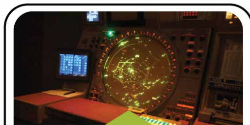
AUTOMATED RADAR TERMINAL SYSTEM (ARTS)
